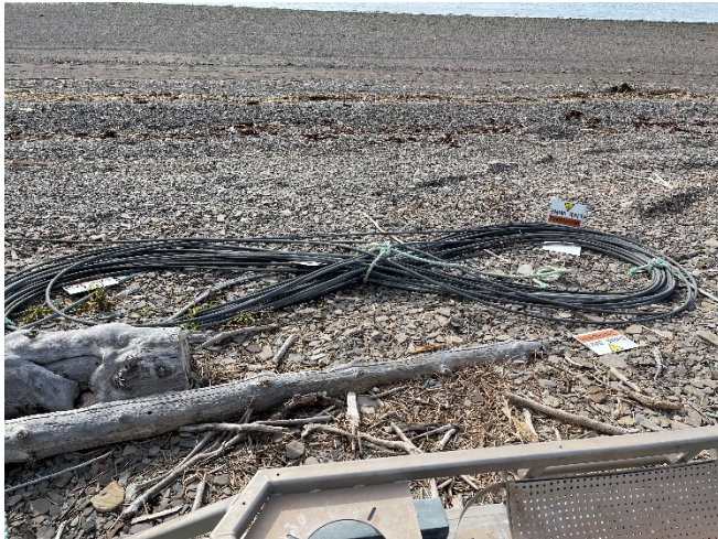
Figure 37: Excess Cable Spooled on the Beach
