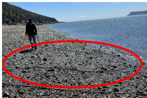
Figure 36: Excess cable on beach after cable lay
